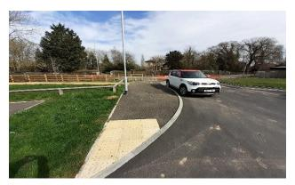
• Agreement to be reached on position of Metal Fencing adjacent to properties as Drawing seems to show 500mm Service Strip, which is now enclosed by Fence.
