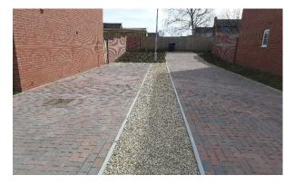
• Slabs & Shingle are required to be changed to Tarmac with Service Strip, righthand side No96, plus lefthand side No102
